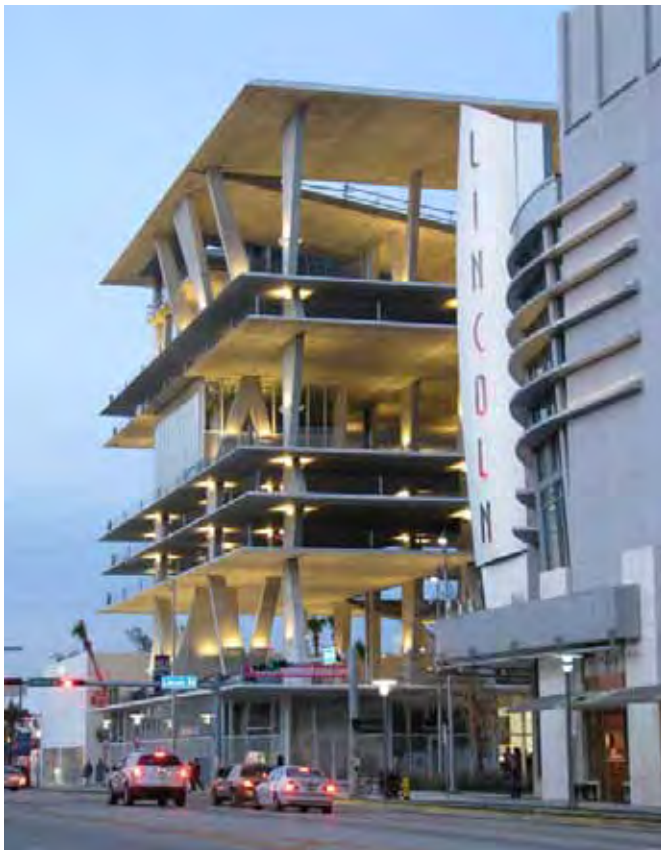
Parking 1111 Lincoln Road, Miami, FL, Herzog & De Meuron
